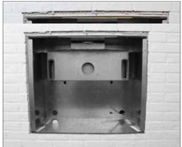
Zero Clearance Box and coaxial flue adapter
