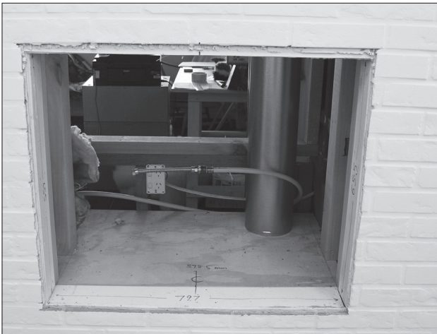
False Fireplace enclosure
