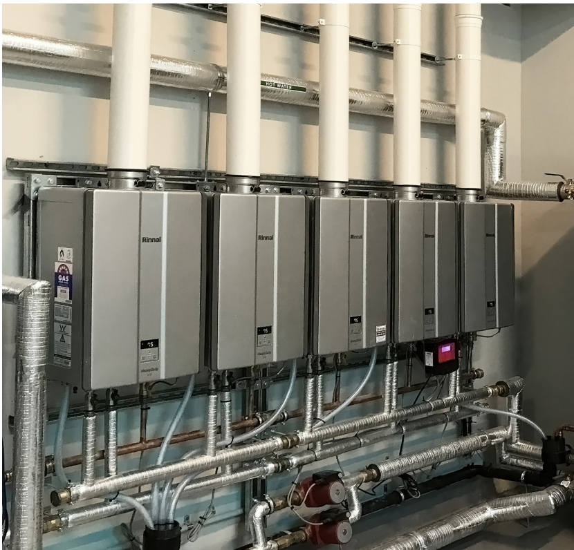
2. Individual flueing per water heater known as co-axial flue
