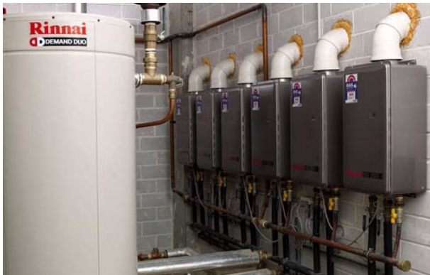
DD6 Internal Flued System
